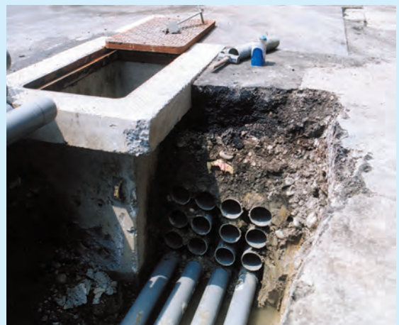
固網通訊工程 Cable net-work communication engineering
